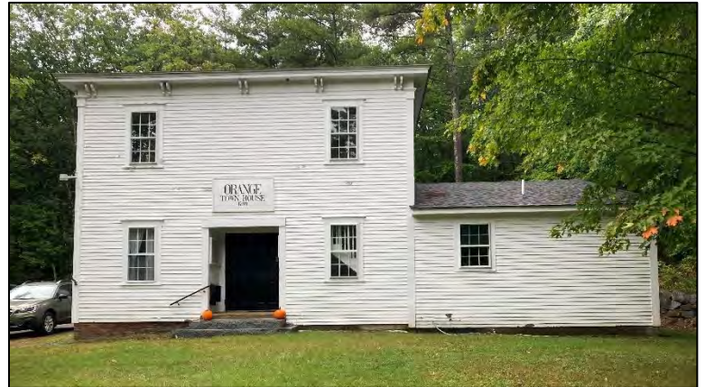
Orange Town House, Rehabilitation - Courtesy Photo
