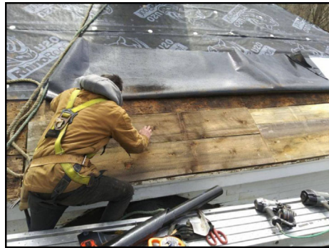
Up close and personal on the Hinsdale House roofing job
